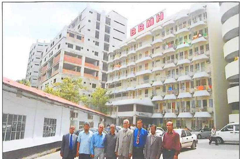
View of BBMH and annex building of BBMH, USTC.
