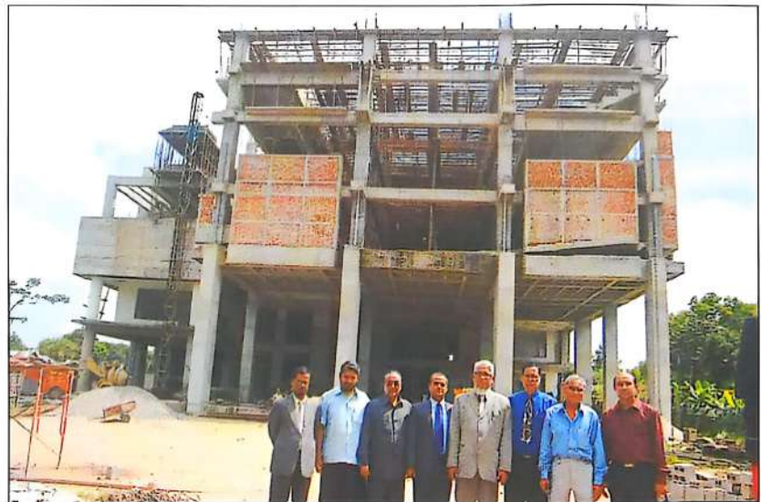
16-storied D-Block, USTC (under construction).
