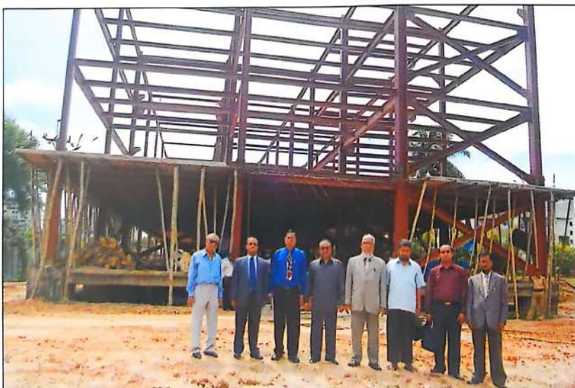
8-storied steel-structure building, C-Block (under construction).
