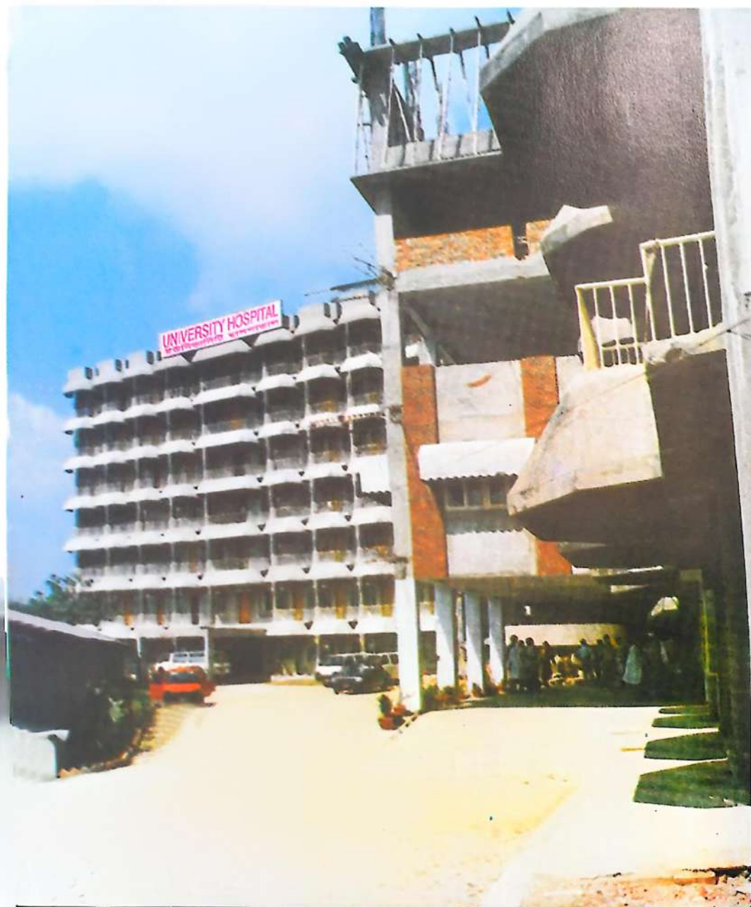
UNIVERSITY HOSPITAL & ACADEMIC BLOCK (5th floor under Construction)
