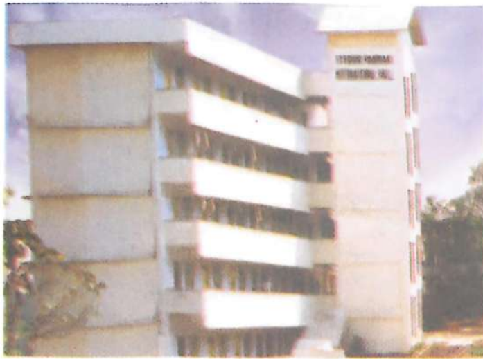
Syedur Rahman International Hall (Accommodation -200) and Executive Block
