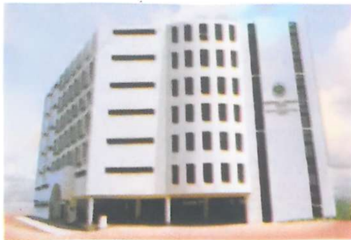
USTC Central Library, Auditorium and International Guest Corner
