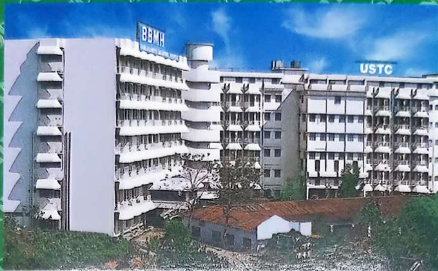
USTC BANGABANDHU MEMORIAL HOSPITAL (BBMH) & ACADEMIC BLOCK
